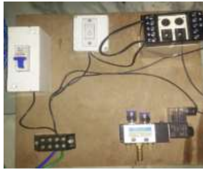
Fig: 4.4-Setup of MCB, Solenoid valve, Bell Switch and cyclic timer
